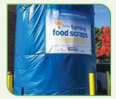
The two Grind2Energy food waste systems on campus collect organic food waste that is eventually transformed into renewable energy and nutrient rich fertilizer after undergoing an anaerobic digestion process. One Grind2Energy system lives at the Tsongas Center Arena.
